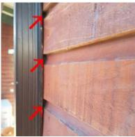
Flashings over windows and door Well fitted flashings. areas:
