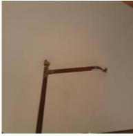
Seismic Strap: Seismic strap not fitted, Requires a seismic strap to be fitted.
