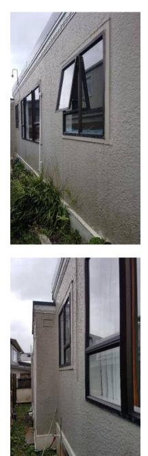
Remedial attention suggested, Damage evident, replacement of damaged area may be the best or easiest option here. This area is a potential moisture ingress risk point. This area may have leaked in the past causing damage to the wall framing which cannot be seen on our visual non invasive inspection. Further investigation is required.
