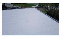
Remedial attention suggested, water pooling and leaks inside found below this area. The roofing material requires further investigation by a licensed roofer to give you the right advice on the degree or replacement, upgrades and costings.
