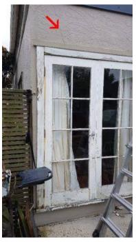
Remedial attention, cracking evident. This area is a potential moisture ingress risk point. This area may have leaked in the past causing damage to the wall framing which cannot be seen on our visual non invasive inspection. Further investigation is required.
