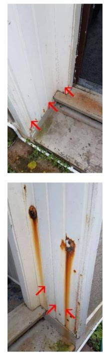
Historical moisture signs evident but no moisture readings of concern were found in this area on the day of inspection. As this is only a non invasive inspection we cannot determine if there has been any damage caused to the framing. Further investigation is required.
