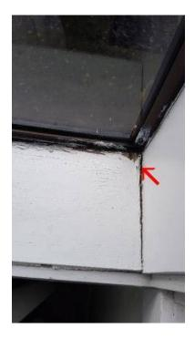
Door types and function standards Hinged door, Not functioning as designed, Remedial attention suggested, Door for this room: adjustment or trim required, door is catching at the top.
