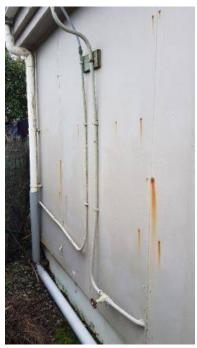
Compressed fiber cement, The cladding may or may not be asbestos, refer to main summery (please read all comments) Remedial attention suggested, Damage evident, replacement of damaged area may be the best or easiest option here.
