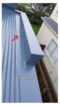
Remedial attention suggested, fully rusted out original flashing, Poorly installed new flashings in this area, This area is a potential moisture ingress risk point. This area may have leaked in the past causing damage to the wall framing which cannot be seen on our visual non invasive inspection. Further investigation is required. The roofing material requires further investigation by a licensed roofer to give costings.
