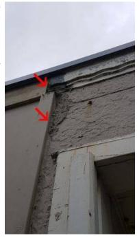
Remedial attention suggested, Damage evident, replacement of damaged area may be the best or easiest option here. Further investigation is required as the condition of the timber is not known, damaged may have been caused within the wall and roof cavity that cannot be viewed on our non invasive inspection.
