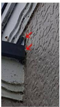
Remedial attention suggested. Poorly installed flashings in this area, This area is a potential moisture ingress risk point. This area may have leaked in the past causing damage to the wall framing which cannot be seen on our visual non invasive inspection. Further investigation is required. The roofing material requires further investigation by a licensed roofer to give costings.
