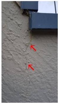
Remedial attention, blown out plaster, this is a sign of moisture ingress. This area is a potential moisture ingress risk point. This area may have leaked in the past causing damage to the wall framing which cannot be seen on our visual non invasive inspection. Further investigation is required.
