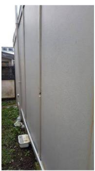
Remedial attention all the sheet fixings are rusted, this is a sign of moisture, further investigation and treatment or replacement is required.
